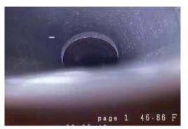
Severe pipe offset ahead, unable to push camera through
