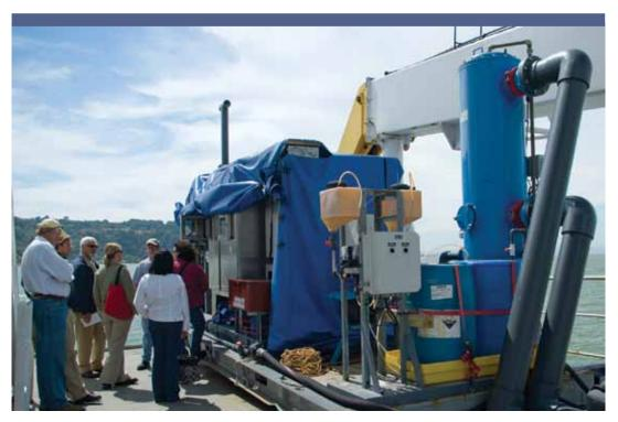
GBF team members and representatives of California State Lands Commission (California's lead ballast water regulation agency) view open-deck installation of the Balpure<sup>™</sup> ballast water treatment system on T/S *Golden Bear*. Image courtesy Lynn Takata, CSLC.
