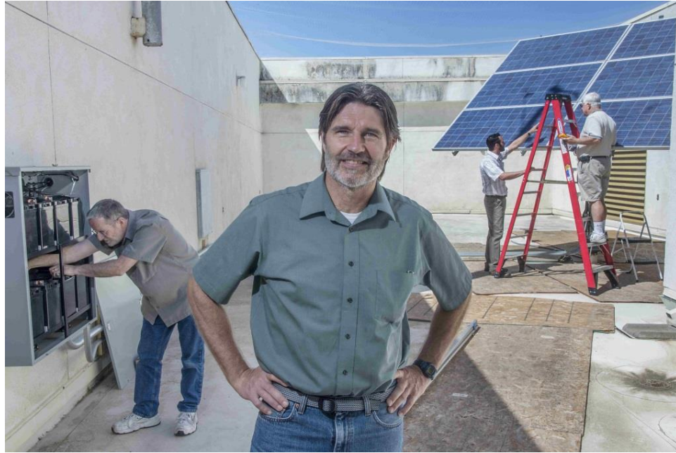
Figure 1. PV array and battery bank in OCNL building roof alcove.
