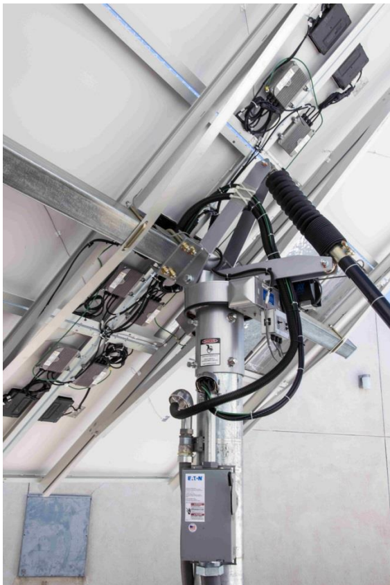
Figure 2. Pole-mount tracking mechanism.
